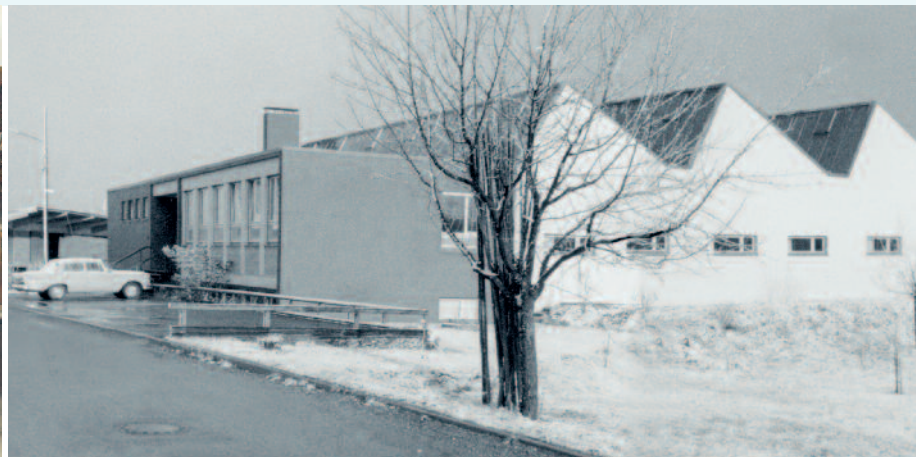
New building 1963 in Weinstadt-Grossheppach
